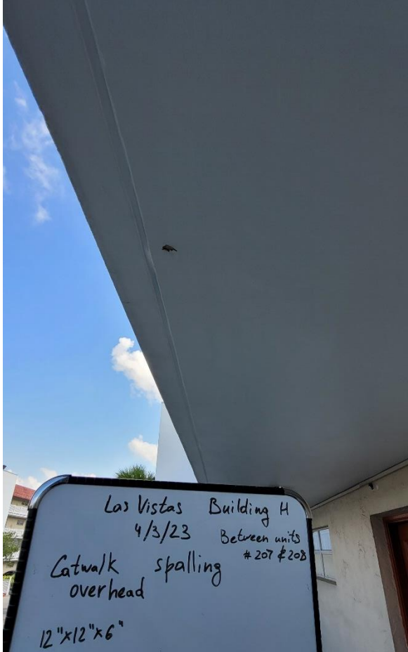
Between Units 207 and 208
