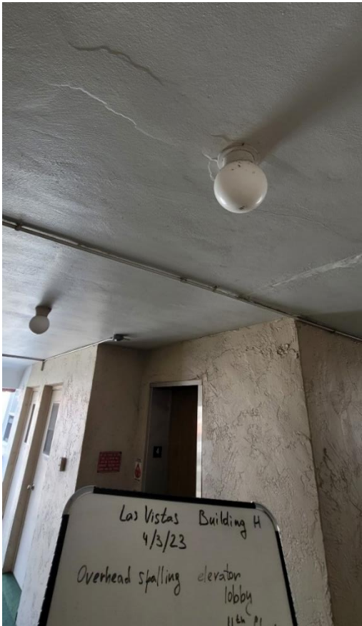
Next to elevator 4 th floor
