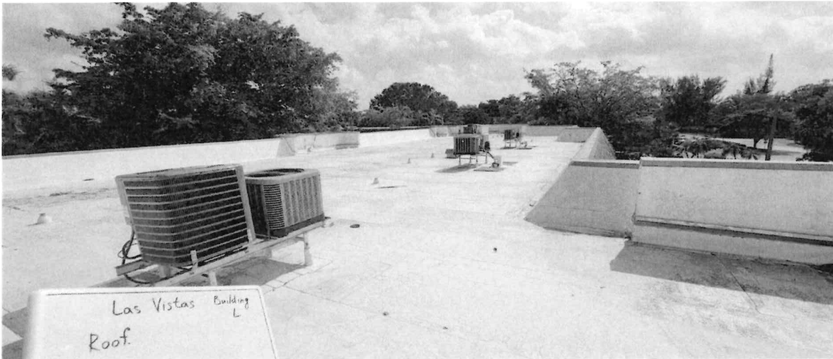
Photo 5: Roof View. No overflows observed.
