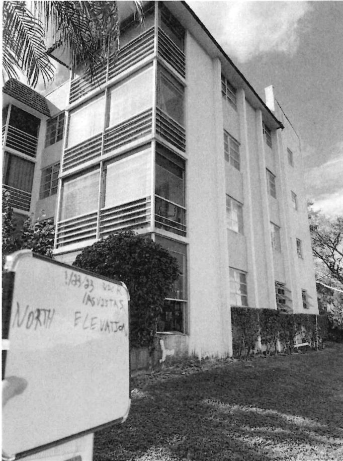
Photo 4: North side view
