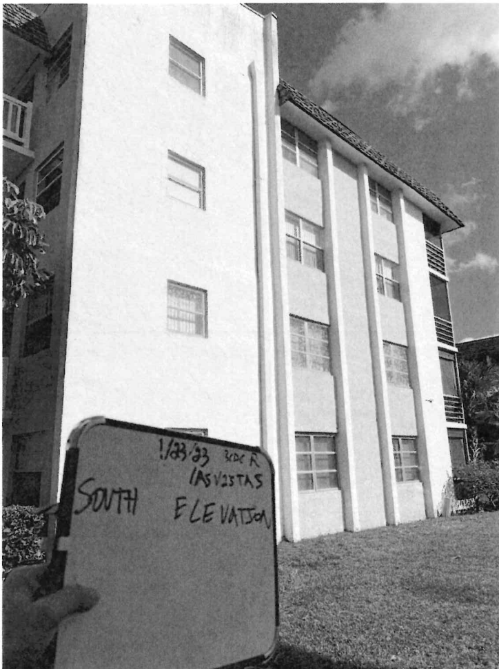
Photo 1 : South Side View.
