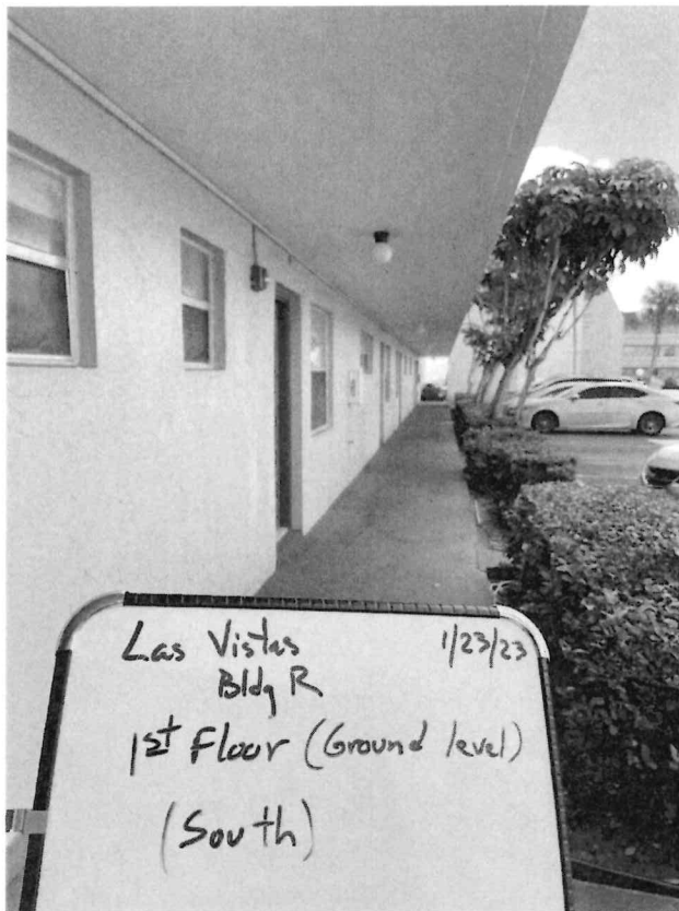
Photo 24: 1st floor ( Ground level ) south.
