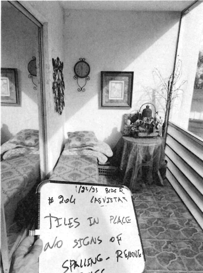
Photo 20: tiles in place no sign of spalling unit 204.
