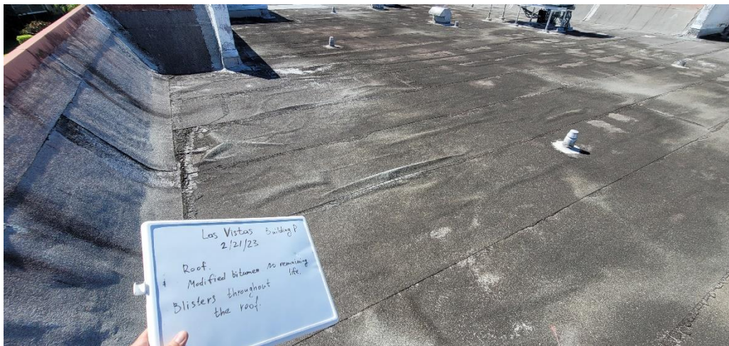
Roof: Blisters throughout the roof. The roof system must be replaced.
