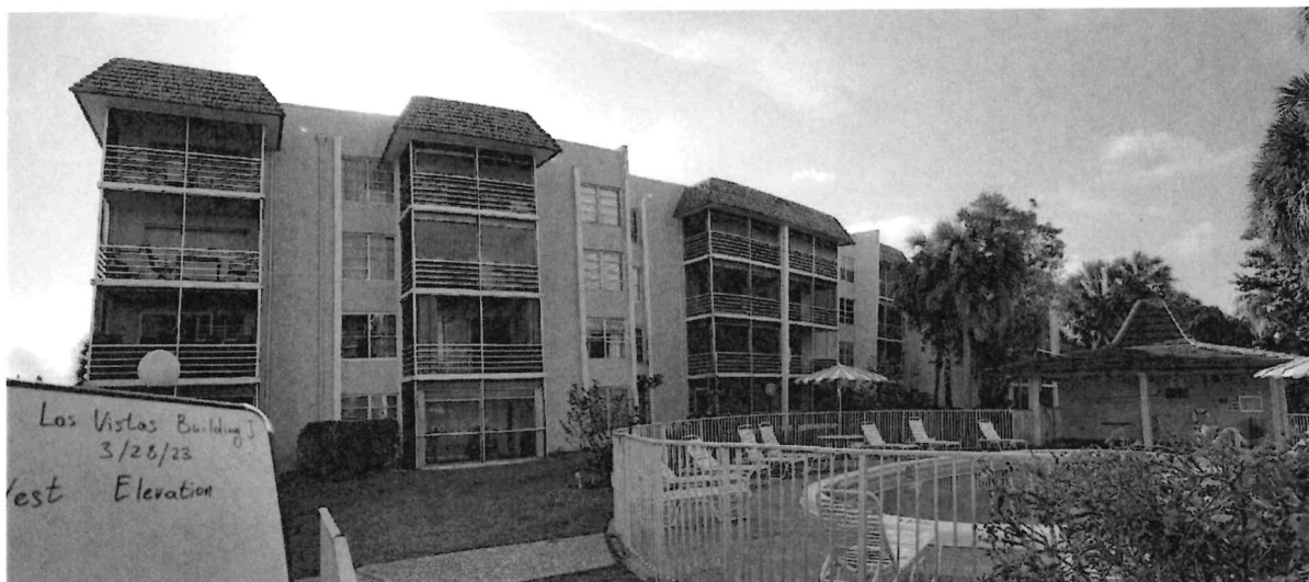
Photo 6: West Side View.
