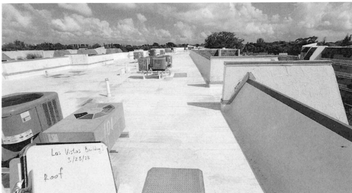
Photo 7: Roof View. No overflows observed.
