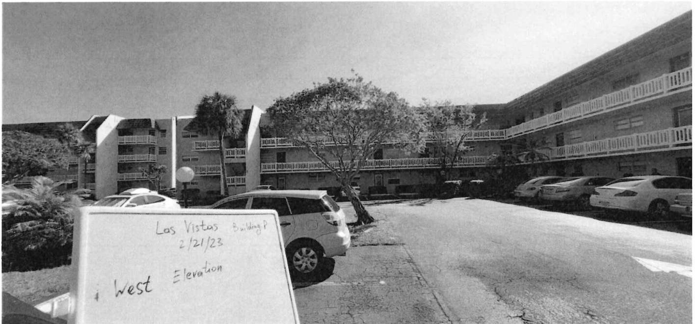
Photo 4 : West Side View.
