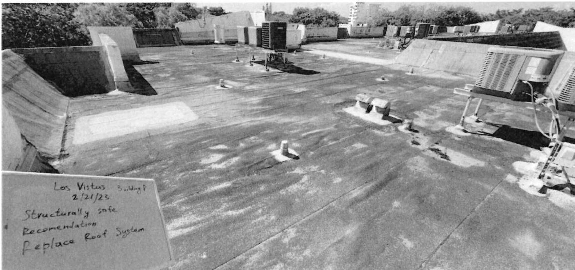
Photo 11 : Roof Structurally safe. Recommendation replace roof system.
