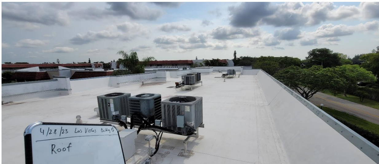
Roof (Single-ply roofing system. Good condition)
