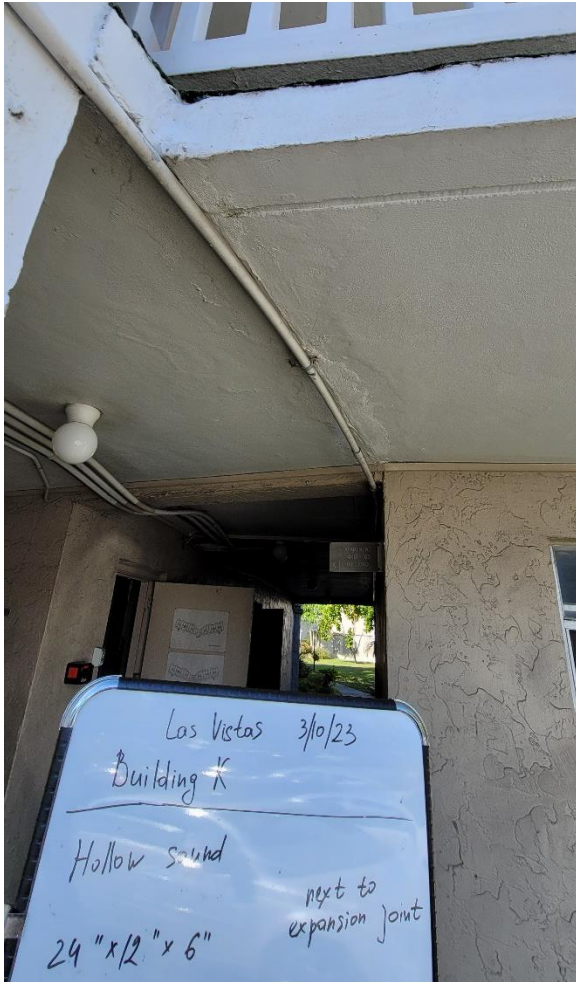
Catwalk next to expansion joint
