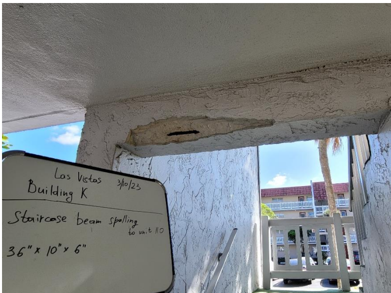
Staircase beam next to Unit 110
