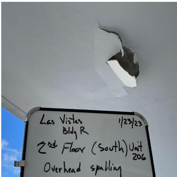
Overhead spalling in front of unit 206
