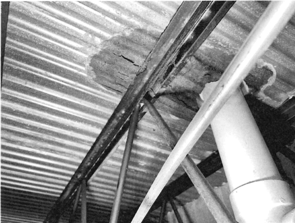
Photo 10 : Meeting room location #1. Observed damaged wood top truss chord and wood deck due to water leaks.
