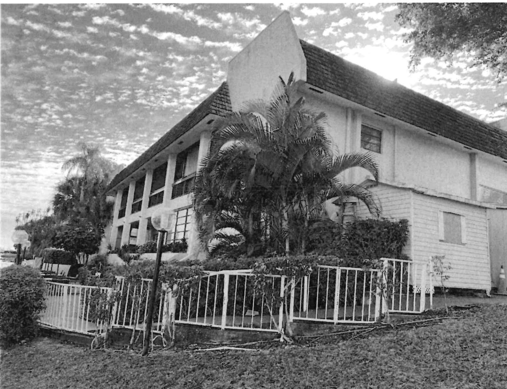
Photo 6: West Side View. Notice aluminum guardrails at balconies.
