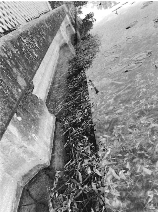
Photo 18 : Sea wall at North side.
