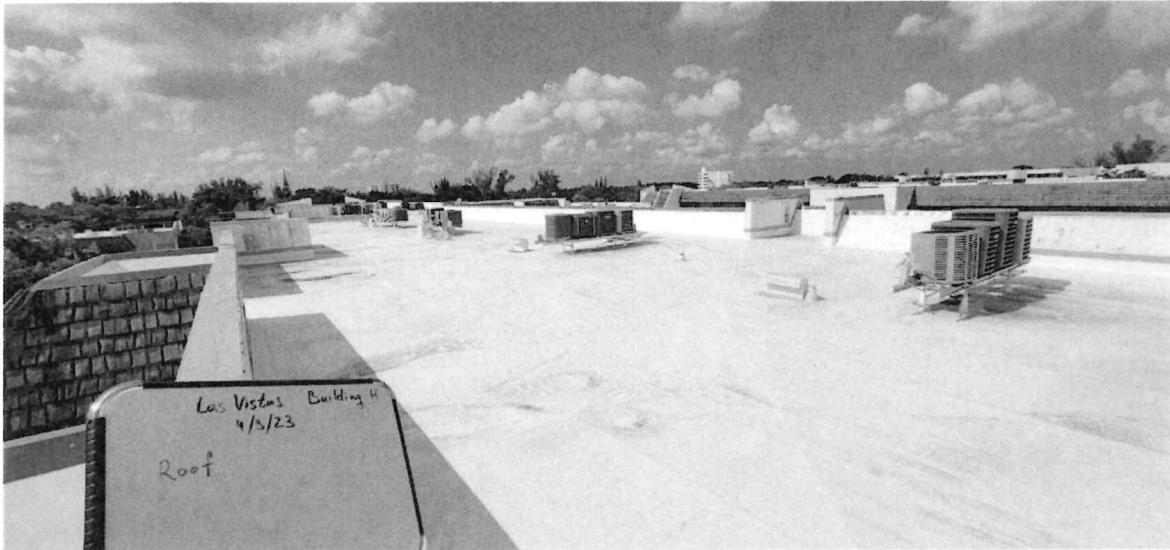
Photo 5: Roof View. No overflows observed.
