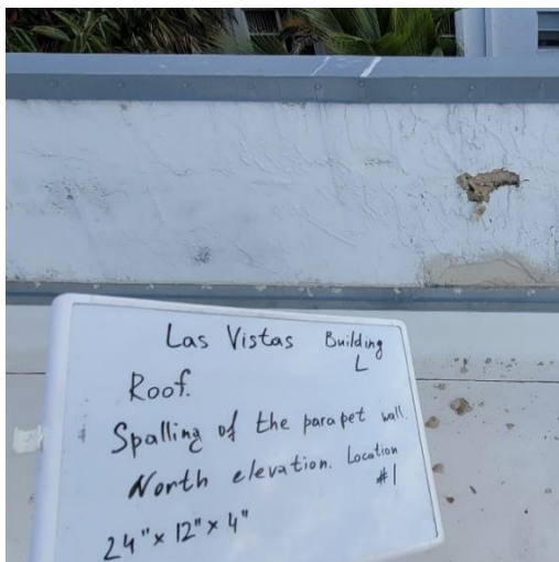
Spalling of the parapet North side
