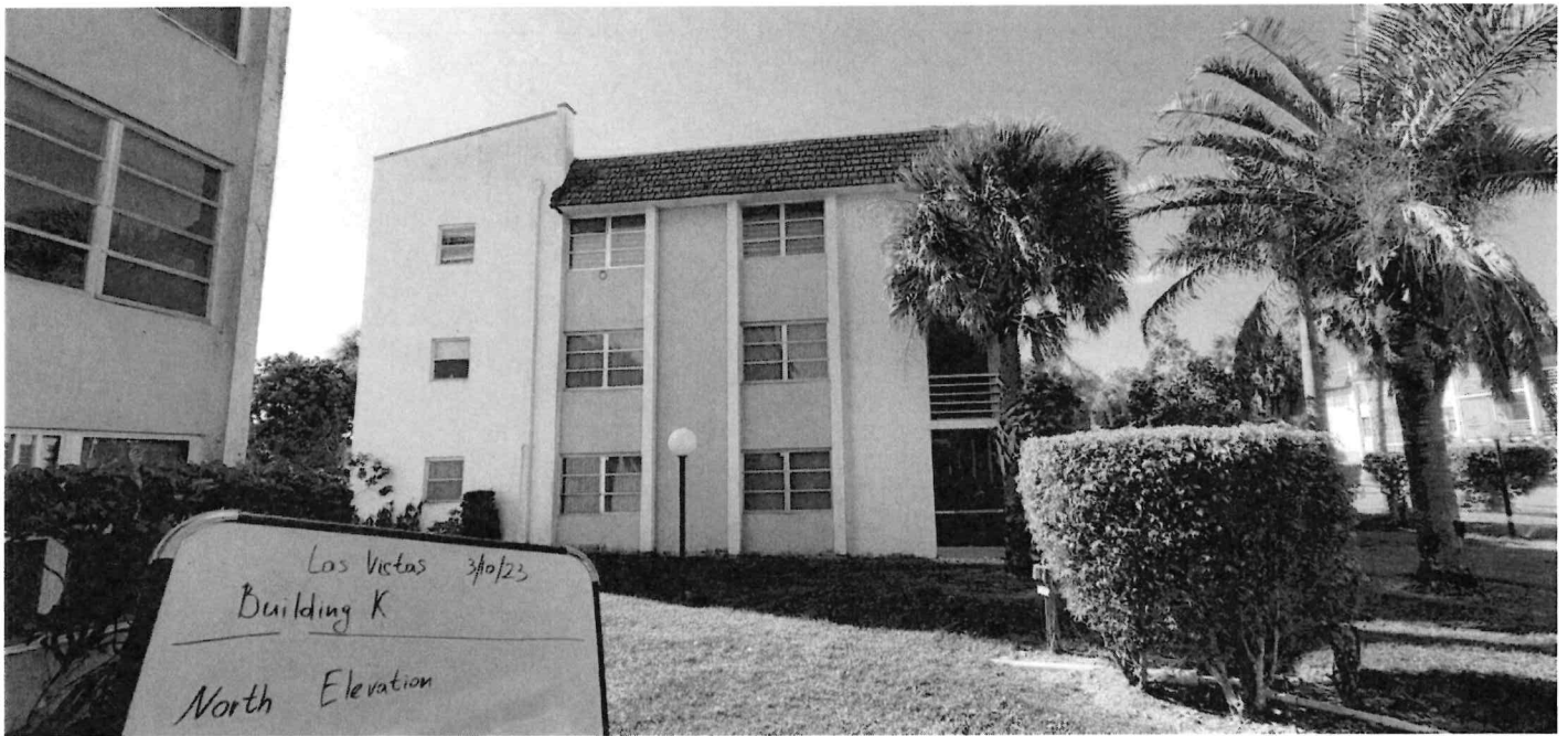
Photo 3: North Side View
