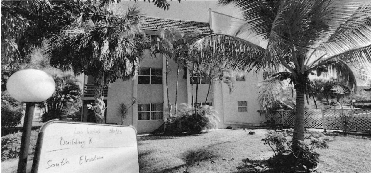
Photo 1: South Side View.
