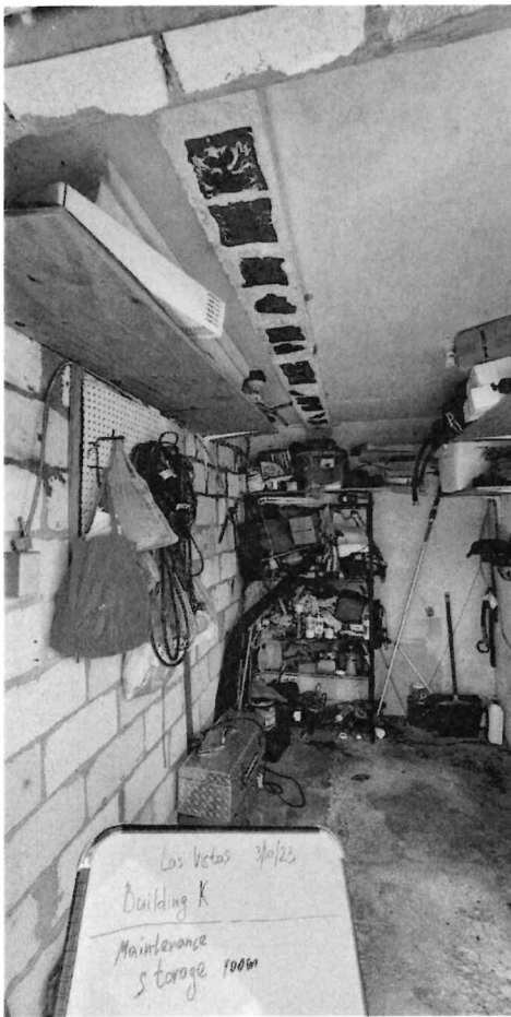
Photo 10: Maintenance storage room
