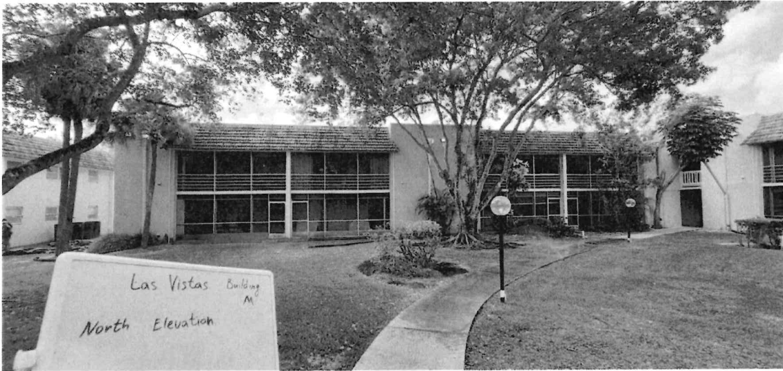
Photo 3 : North Side View.
