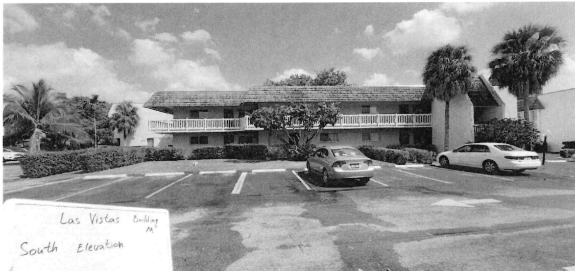
Photo 1: South Side View.
