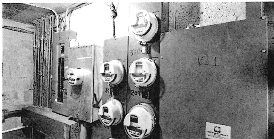
Main disconnects and metering equipment.
