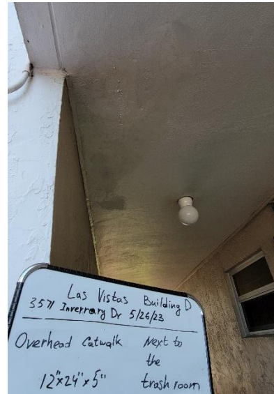
Next to trash room
