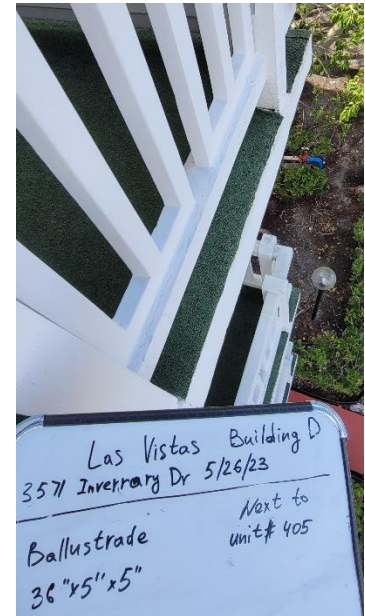
Balustrade next to Unit 405
