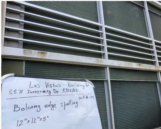
Balcony slab Unit 109
