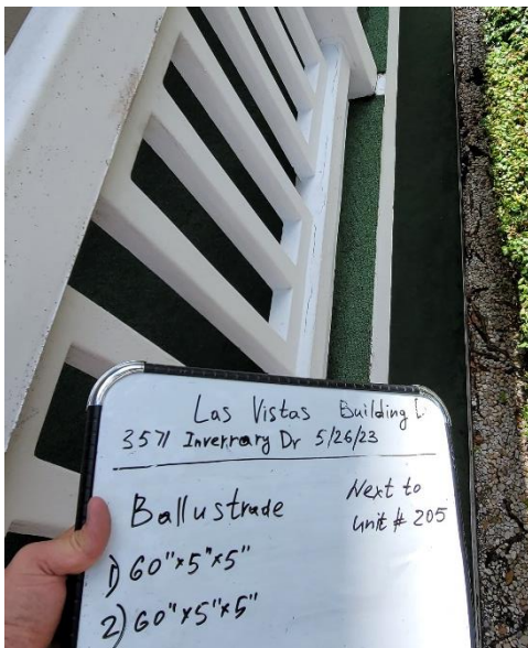
Balustrade next to Unit 205
