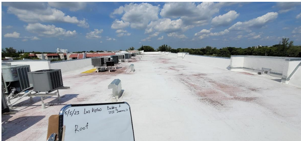
Roof (Single-ply roofing system. Good condition)
