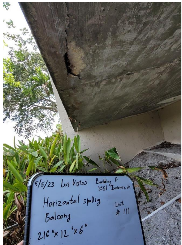
Balcony slab Unit 111
