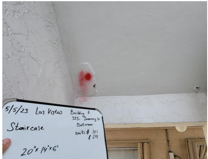
Staircase between Units 101 and 201
