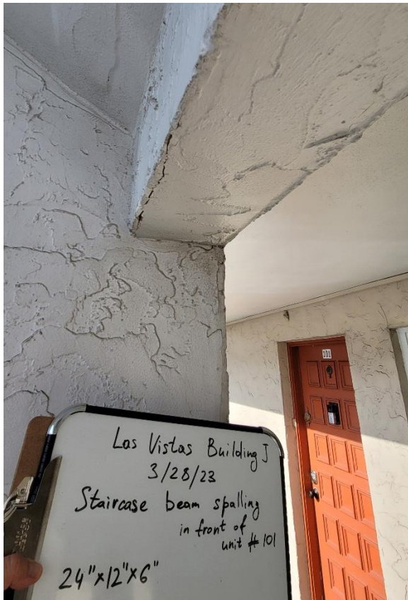
Staircase beam in front of Unit 101
