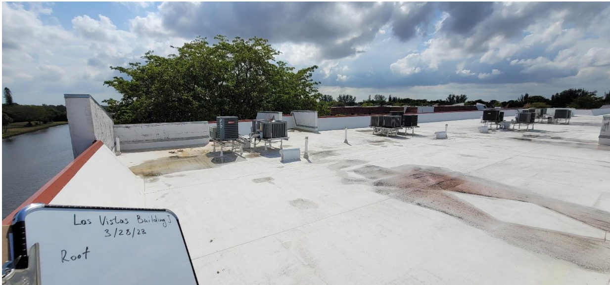
Roof (Single-ply roofing system. Good condition)
