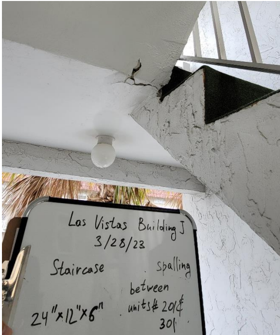
Staircase between Units 201 and 301
