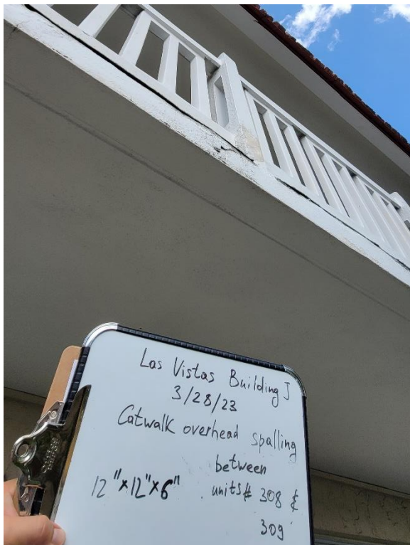
Between Units 308 and 309
